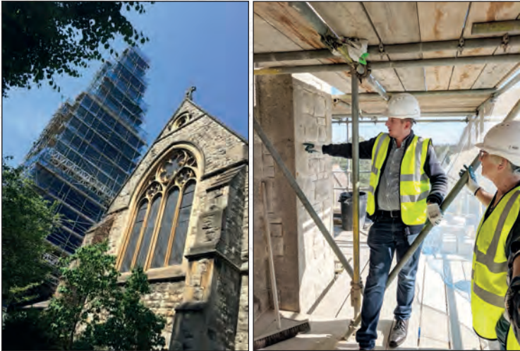
Wreathed in scaffolding, St Matthew's steeple. Right: Site foreman Jerry Sojka points out to intrepid climber Johnnie Byrne where a stone has been replaced
