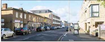
How Brighton Road will appear after Brandon Tool Hire and the Museum of Futures are demolished, like Elton Park Motors, to make way for new homes.
